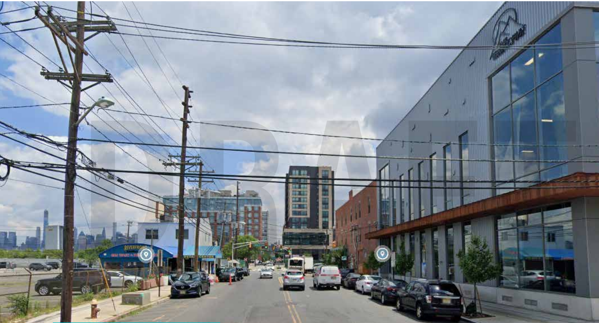
15TH STREET LOOKING TOWARDS HUDSON RIVER
