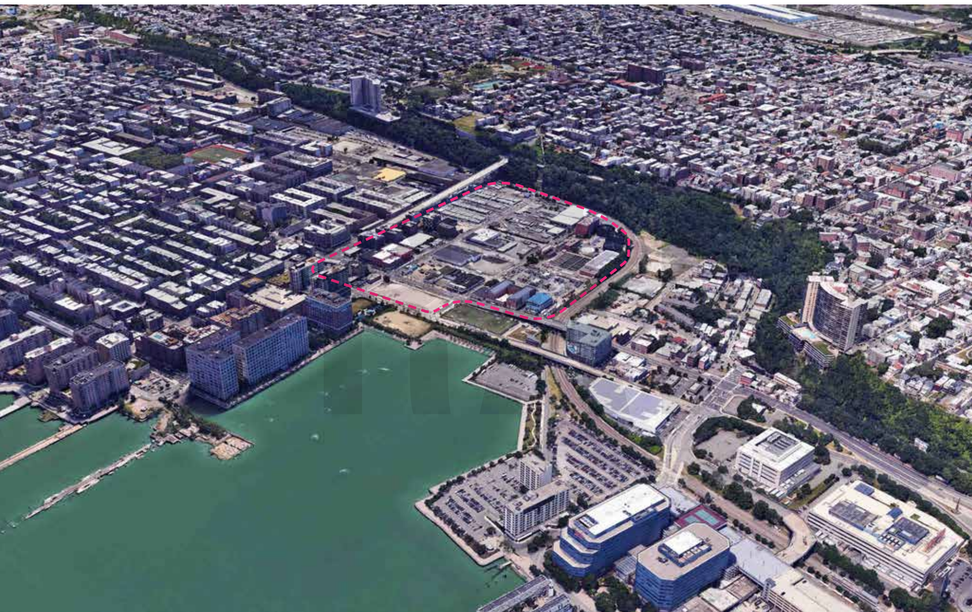
^ FIGURE 3. AERIAL VIEW OF THE NORTH END REHABILITATION AREA FROM THE HUDSON RIVER
