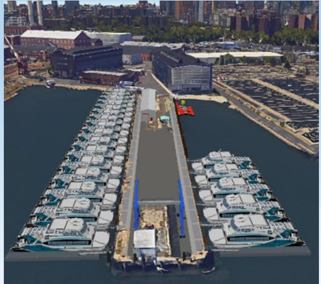
Example: East River Ferry Facility (under construction at Brooklyn Navy Yard)
