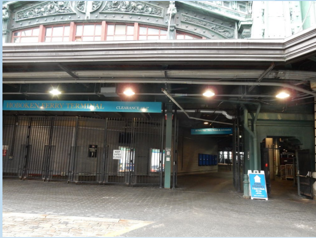
Warrington Plaza Access 11' 2" Vertical Clearance
