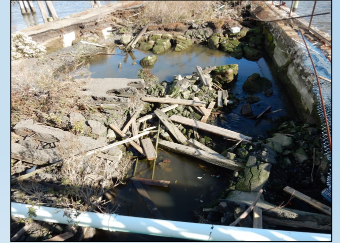
Interior Conditions of South Pier (western end)
