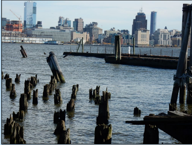
Remaining South Pier (eastern end)
