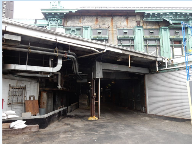
Access from South Side of Platform
