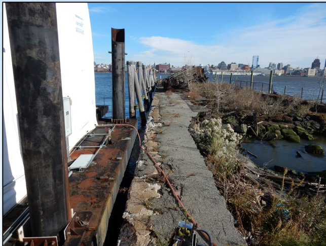
North side of South Pier (western end)
